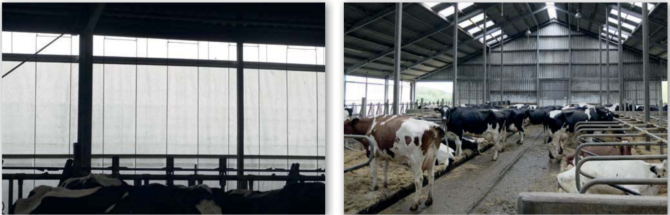
Figure 5: Closed and dirty ventilation curtains (source: Pelzer)
